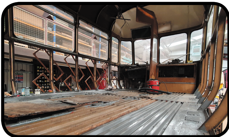
DRB Keighley end floor restoration - Photo: Richard Jones
