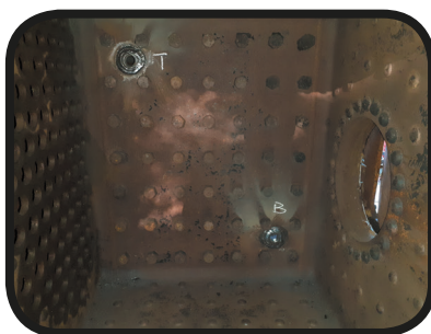
Repairs to the fusible plug holes in the firebox
