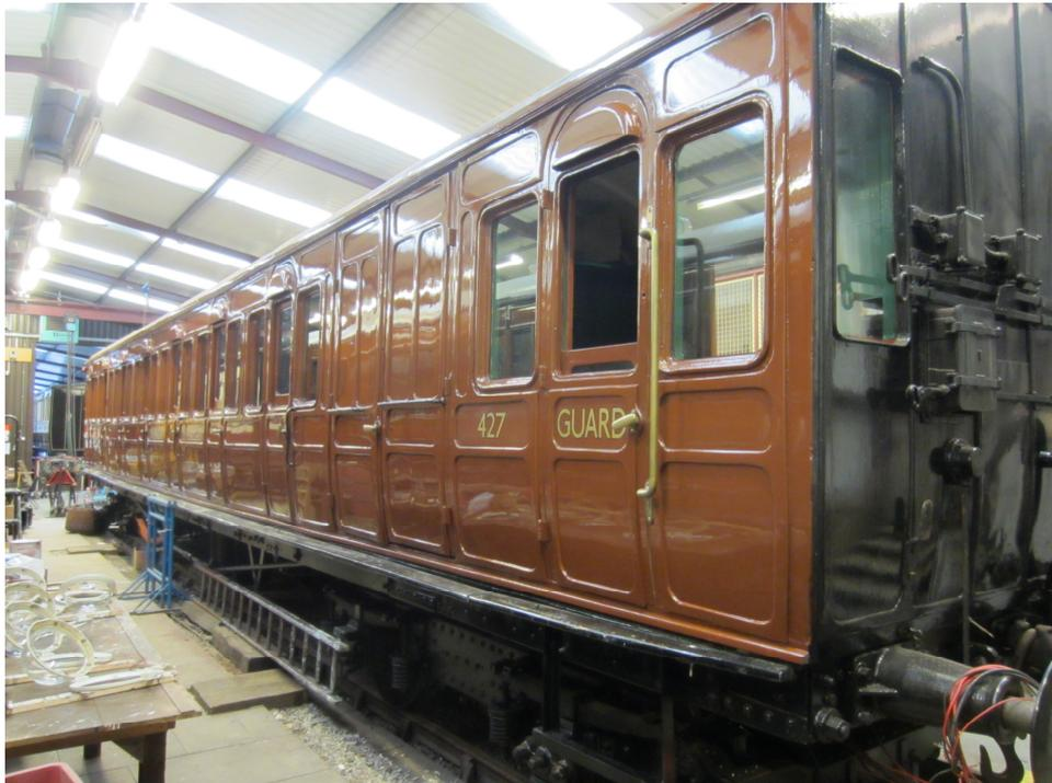
The body has now been re-seated on to its rebuilt underframe and is now structurally in very much better order than it will have been for several decades past. Following his many weeks of work on the underframe Chris is now re-painting and varnishing the body, to good effect (as shown to the left). This will complete the major programme of work on this coach. We take the opportunity to congratulate Chris on his significant achievements here.
